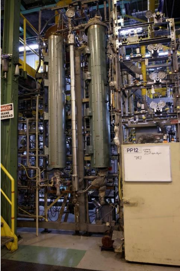
0.5 barrel (80 L)/day hydroprocessing unit with 2 reactors and on-line distillation
