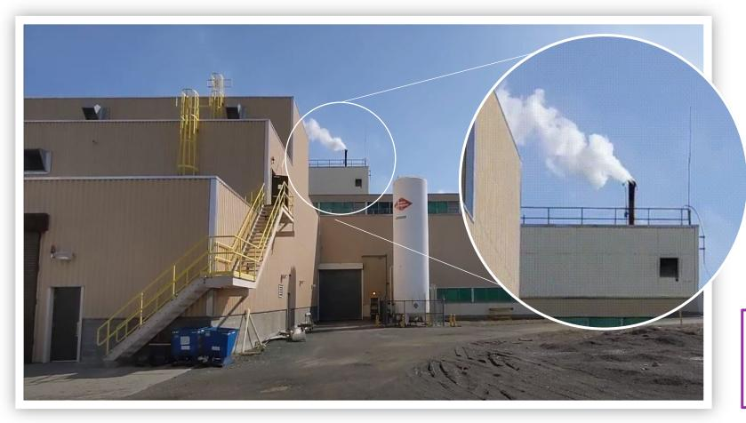
Byproduct hydrogen is produced during industrial processes and typically vented into the air.
